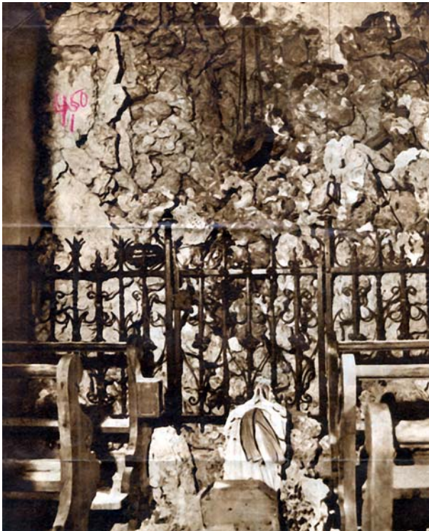
Fig. 5 The “Antonius Chapel” in Sarnen was built in 1646. The Earthquakes of 1964 destroyed a precious relief. (Allgemeine Volkszeitung 1964)
