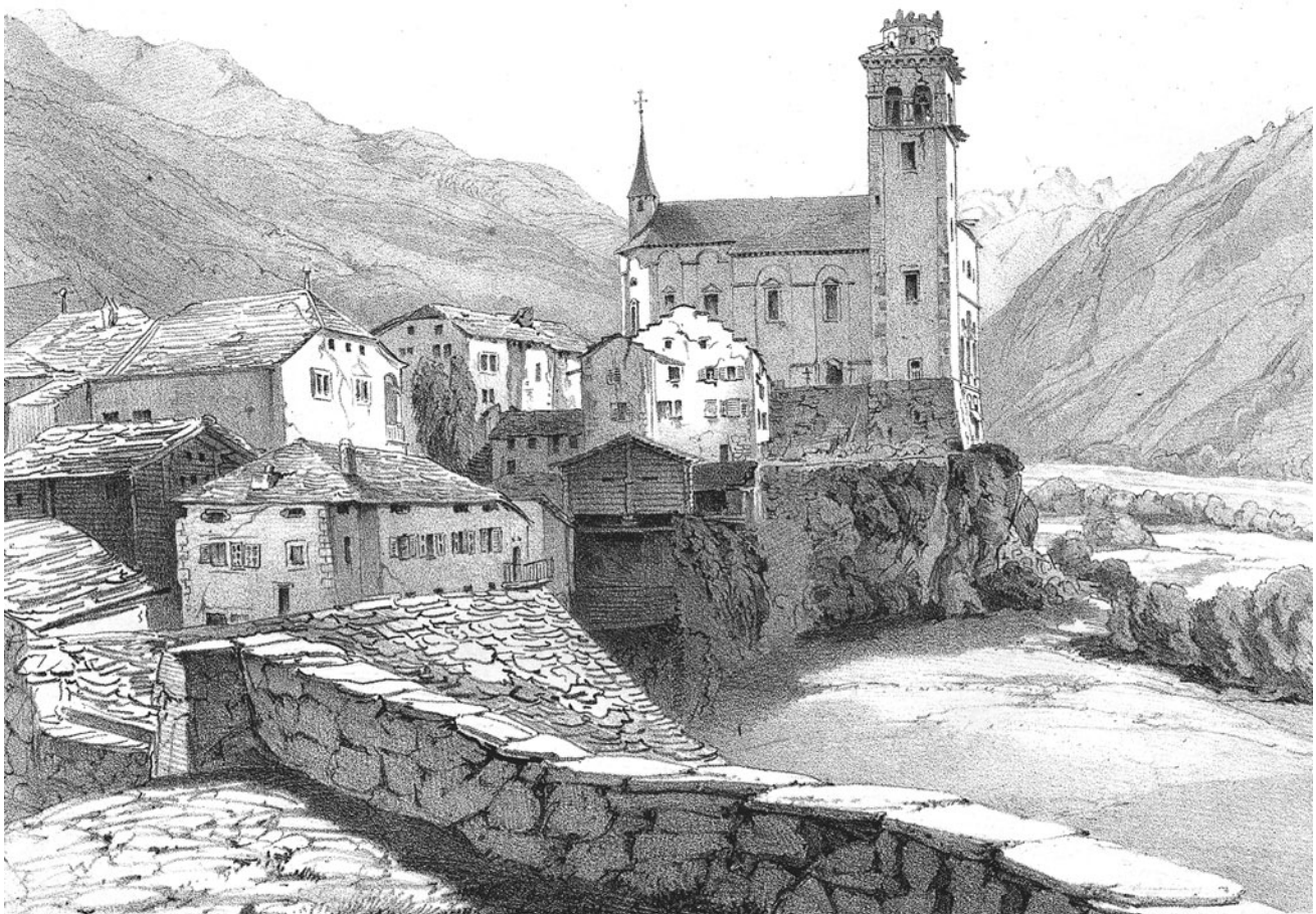
Fig. 5 Visp and the Martinskirche with the tower damaged by the 1855 event (Heusser 1856)
