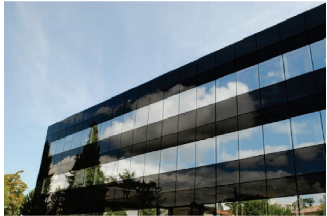
Fig. 34: Rhône-Alpes area (France): PV façade with micromorph thin-film PV panels of 1.10 \times 1,30 \text{ m} each (ou bien: 1.4 \text{ m}^2 ) (Surface: 130 \text{ m}^2 ; Energy output: 738 kWh; System provider: Pramac; Façade: Face InTec, 2011)
