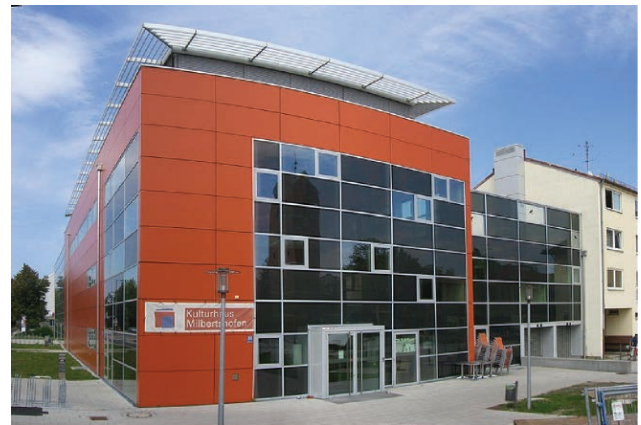
Fig. 31: Kulturhaus Milbertshofen (Germany): façade with black micromorph and semi-transparent thin-film modules (Energy output: 3 kWp), RPM-Architekten, System provider: Voltarlux, 2008)
