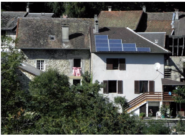
Fig. 2: Typical non-integrated European PV roof-installations (1990s–today)
