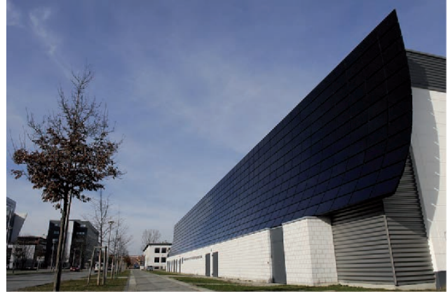
Fig. 15: Ferdinand-Braun-Institute, Berlin: 732 dark CIS modules designed as a curved façade (Surface: 640 m 2 , Energy output 39 kWp, System Provider: Sulfurcell Solartechnik GmbH, 2007)
