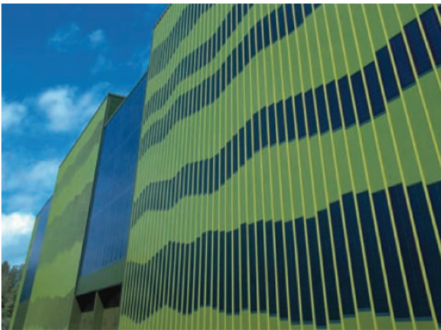
Fig. 37: The Thyssen-Krupp Steel building, Duisburg (Germany): Colourful rendering obtained by coloured steel façade elements (Product: ReflectionsOne) and vertically integrated common Si-solar panels (Surface: 1000 \text{ m}^2 ; Energy output: 51 \text{ kWp} ; Colour Design: Friedrich Ernst v. Garnier, Studio für Farbentwürfe; Architects: Czerny-Gunia, Essen; System provider: ThyssenKrupp Solartec, 2002)
