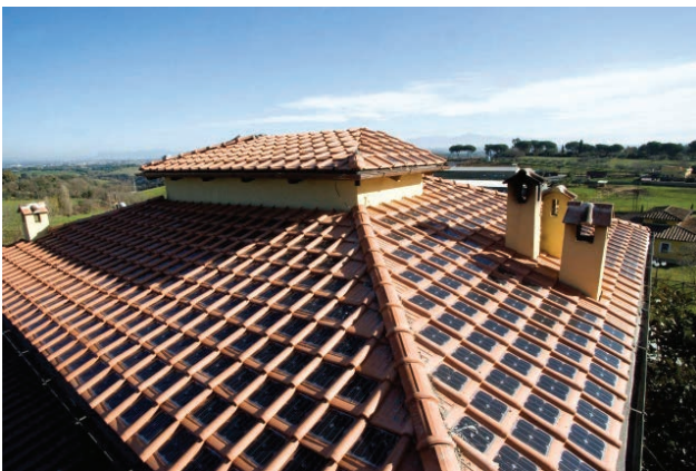
Fig. 27: Solar tiles solution in Italy to meet with Mediterranean roof tradition (System provider: Tegola Solare)
