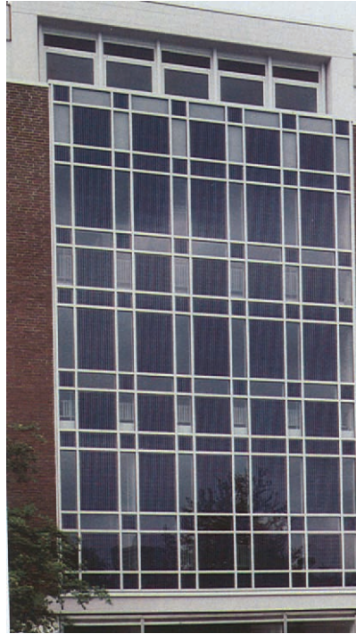
Fig. 3a: Public Utilities Building (Stadtwerke), Aachen (Germany): First façade ever (1991) embedding c-Si wafers into insulation glass (Surface: 37 m 2 , Energy output: 4,2 kWp, Architect: Georg Feinhals, System Provider: Flabeg Solar; Source: Hermannsdörfer/Rüb: Solardesign, 2005)
