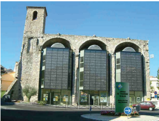
Fig. 6: Building of the Tourist Office in Alès (France): integration of three PV façades into a listed sixteenth-century building (Surface: 100 m 2 , Energy output: 9,5 kWp, Architect: Jean François Rougé; System Provider: Photowatt, 2001)
