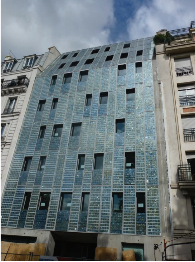
Fig. 41a: Building at Quai de Valmy 179, Paris (France): seven storey façade covered with 130 customized emerald-green multicrystalline Si panels (Surface: 173,6 m 2 ; Energy output: 17 kWp; Architects: Emmanuel Saadi and Jean-Louis Rey, System provider: Sunways AG, 2011)
