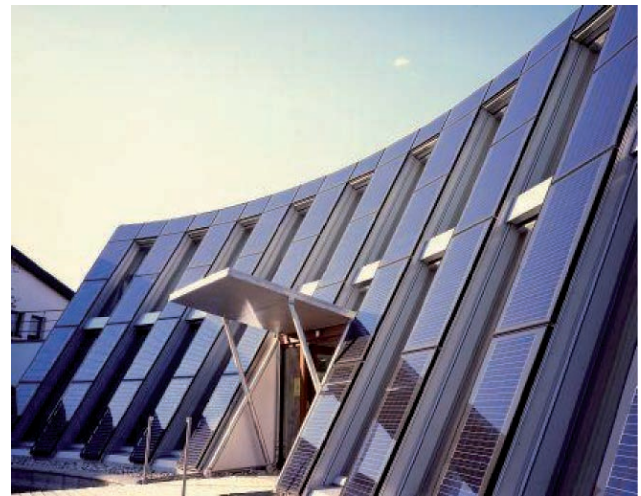
Fig. 30: Juwi Head Office, Bolanden (Germany): ideal façade inclination with large-scale PV modules to harvest a maximum of solar energy (Surface: 70 m 2 , Energy output: 7.2 kWp, System provider: Schüco International KG, 2004)
