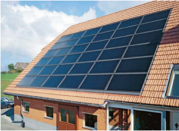
Fig. 18: Typical framed in-roof installation, Sumiswald (Switzerland): the installation achieves a homogeneous appeal through the fact that both, the frame and the modules, share the same colour.
