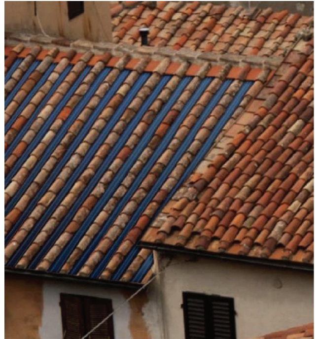
Fig. 28a: Solution by vertical installation of PV panels on Mediterranean roofs (System provider: Hemera)
