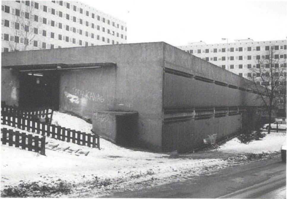
Figure 10: Parking deck in Haugenstua in Oslo.
