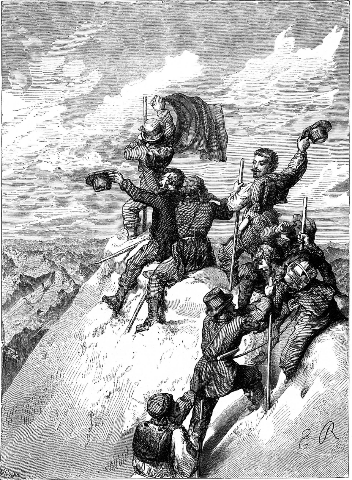
ON THE TOP OF THE WETTERHORN.
