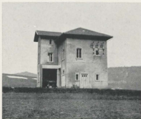
Môtiers: station principale de transformation.
