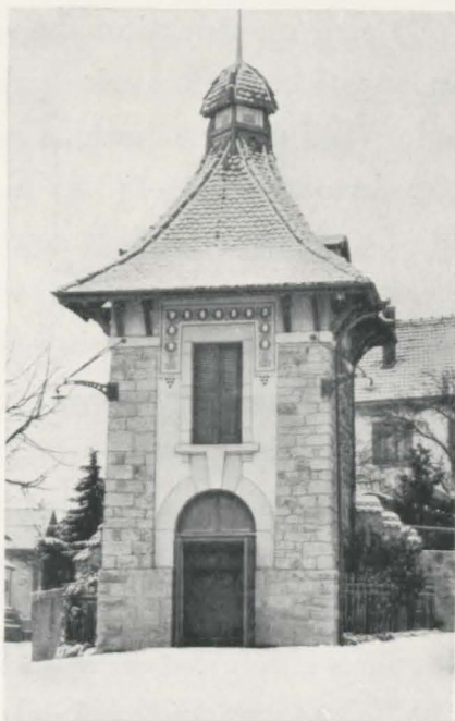
Station de transformation.
