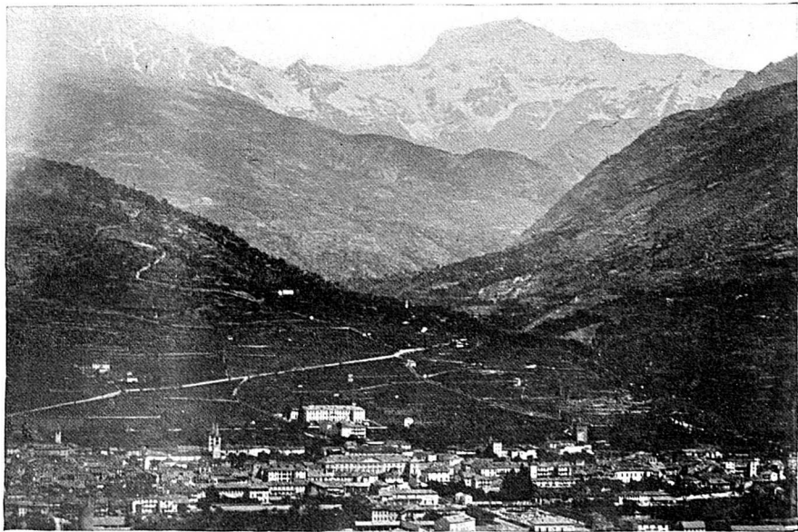
AOSTA — GENERAL VIEW.
