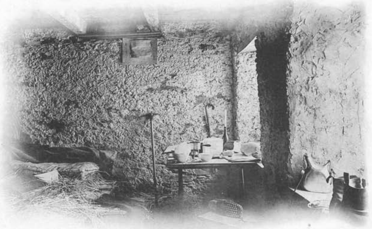
Interior of the hut on the Cervin.
