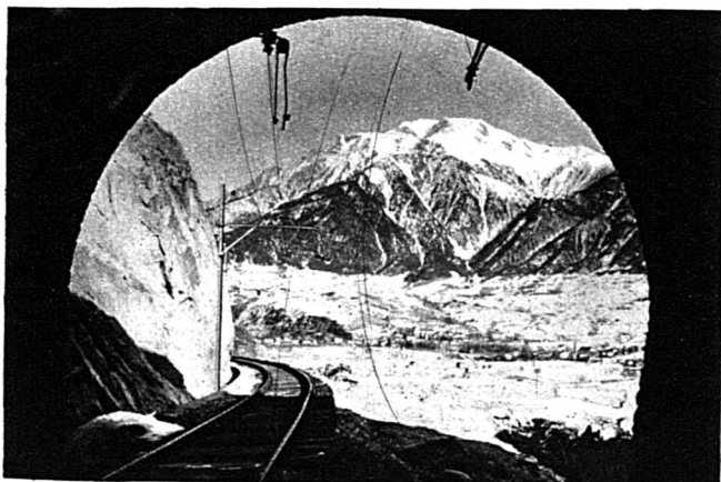
Tunnel of Mundbach-Brigue.
