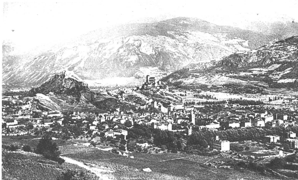
SIGN. -- GENERAL VIEW.
