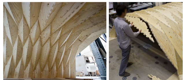
Fig. 8 The MTSJ joints have already been successfully applied to more complex assemblies, where the joint angles \theta_1 , \theta_2 and \theta_3 are not zero (Robeller et al. 2014).
