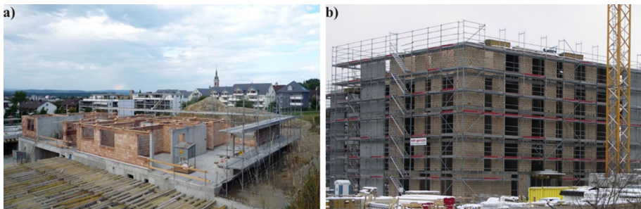
Fig. 1 Examples of new buildings with RC and URM walls in Switzerland (Photos: Thomas Wenk)
