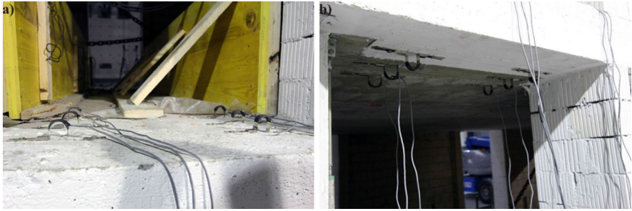
Fig. 40 Omega gages of “Location B”: top face of the slab (a) and bottom face (b)
