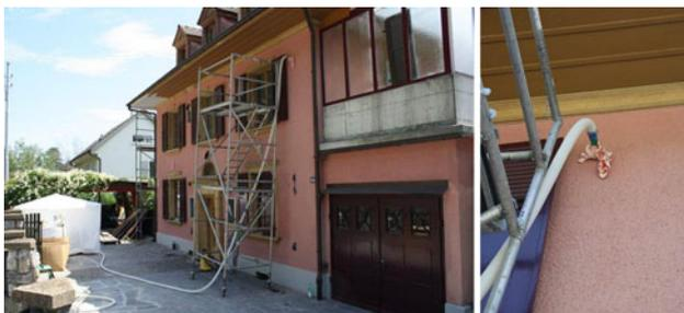
**Fig. 20** Cavity wall insulation with aerogel granulate in Biel, Switzerland. View of the renovation site (*left*) and zoom on the injection hole (*right*)
