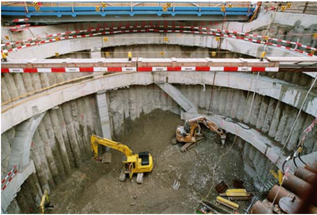
Fig. 5 Tunnel-gate shaft (see Fig. 4, section A–A'). The shaft reaches down to the bedrock
