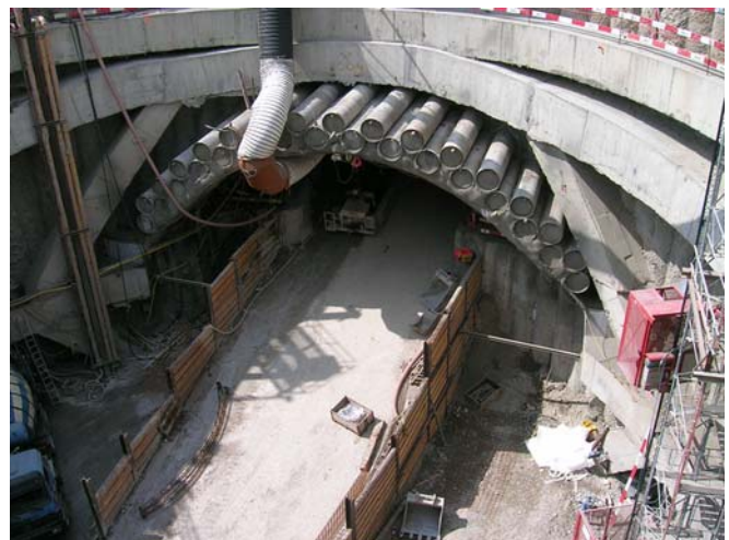
Fig. 6 From the tunnel-gate shaft the highway access and exit roads to the main tunnel are excavated using the “micro pile” mining technique
