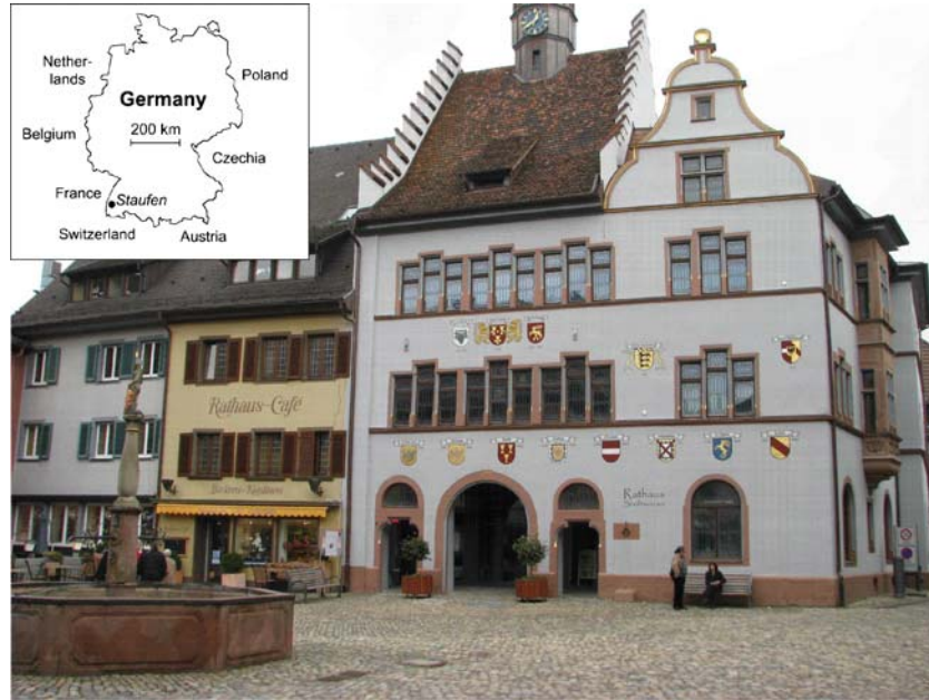
Fig. 1 Location of the town of Staufen and impression of the historic town hall in the city centre
